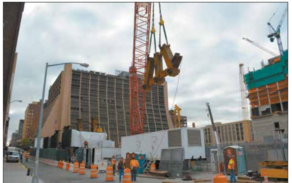
The 750 ton crane slowly raises and swings the column to the Eastern Rail Yard platform, one of two platforms that will support three high-rise offices and residences.
