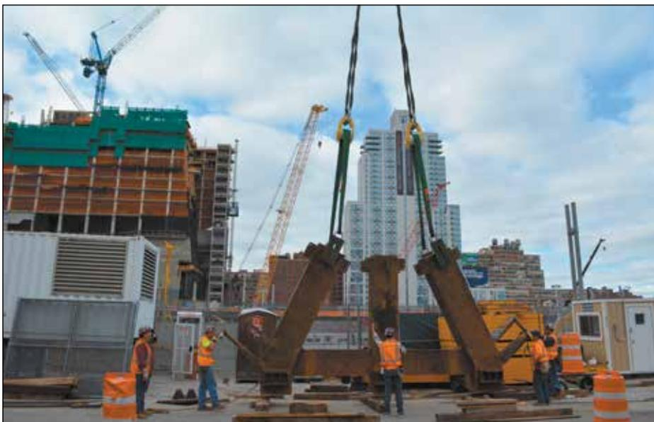
Manitowoc crane equipped with I&I slings and Equalizer Blocks uprights a 45 ton section of A-frame column for platform designed to support skyscrapers at Hudson Yards in Manhattan.
