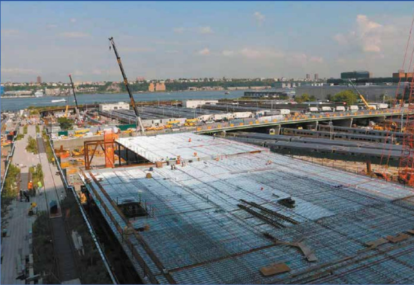
Eastern Rail Yard platform consists of precast concrete slabs on steel framework supported by massive columns that in turn bear on concrete-filled caissons drilled to bedrock.
