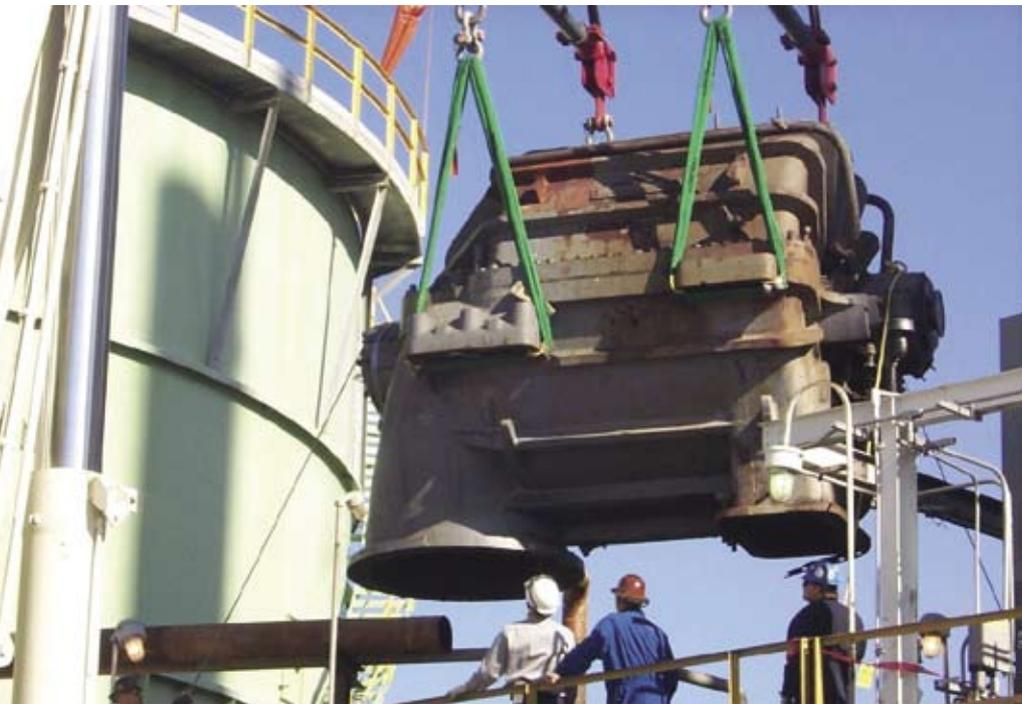
The slings lifting this refinery compressor are shown with cut protection (along bottom with Cornermax Pads) and secondary bearing point/abrasion protection (left sling).
