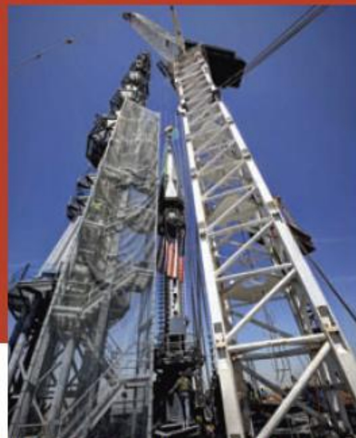
The final spire section was lifted to the roof of the building on May 2 and was erected to its final height on May 10.
