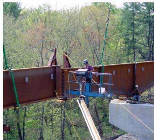
The CornerMax Sleeve is made from a heavy duty weaving process using 100% Dyneema high performance fiber that creates a product with very high cut resistance. Above, the Cornermax Sleeve used during an aerial connection
