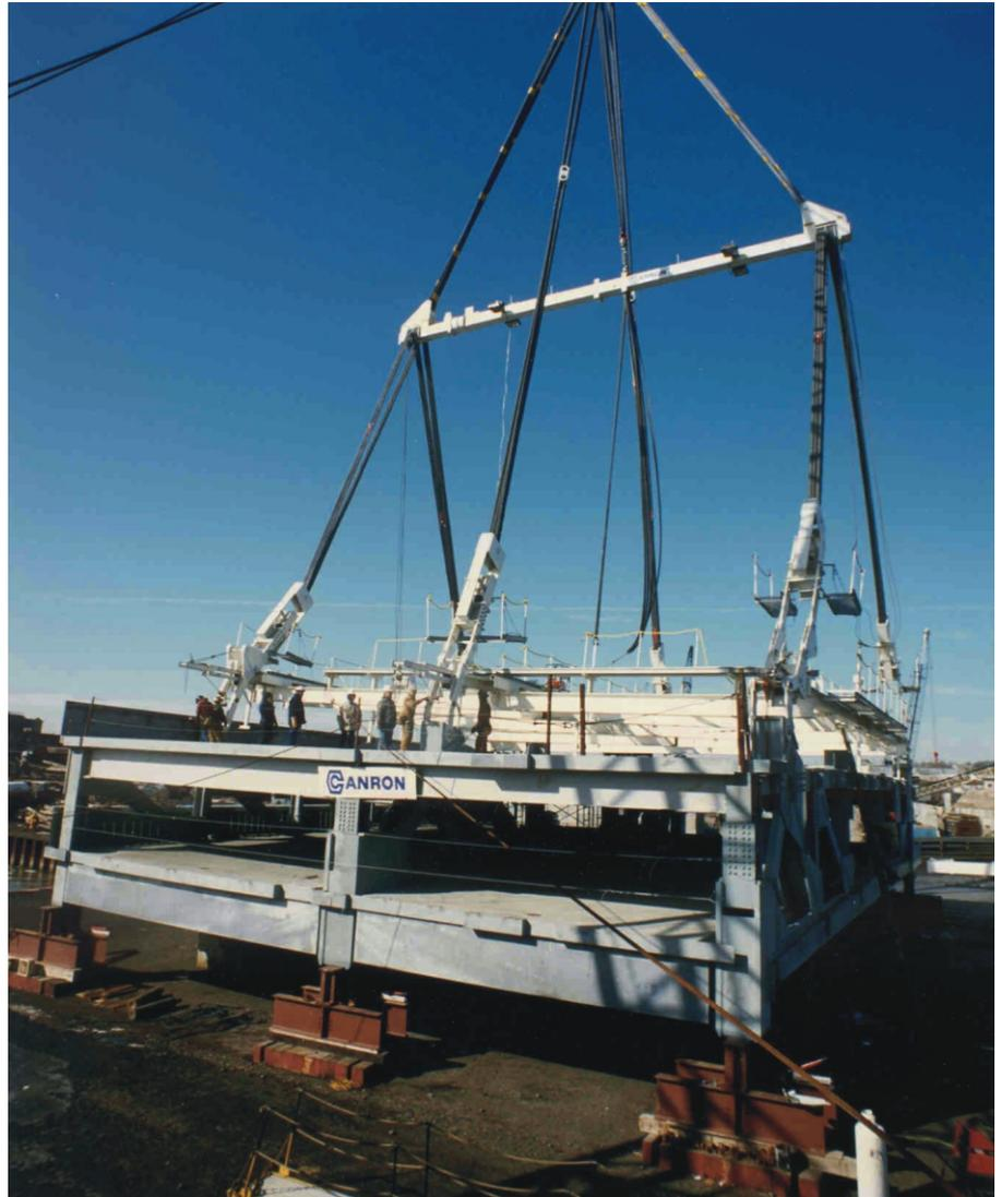
**If wire rope slings had been used for this 760 ton lift, they would have added approximately ten additional tons to the load. Since this lift was made back in 1994, several more in the 1,000 ton range have been safely accomplished.**
