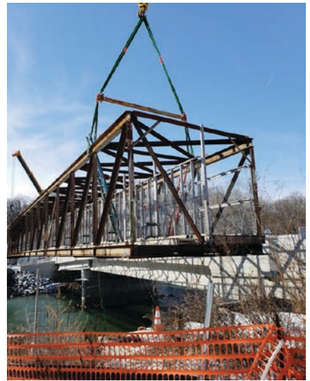
Removal of Pedestrian Bridge, Feb. 14, 2019
