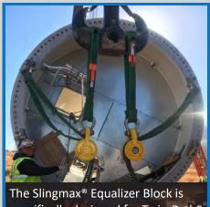
specifically designed for Twin-Path® slings and is the perfect solution for unbalanced loads or tilt-up applications while uprighting wind towers.
